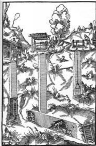
THREE VERTICAL SHAFTS, BY WHICH THE FIRST, A, FROM THE MOUNTAIN SIDE, THE SECOND, B, REACHED THE TUNNEL; BY THE THIRD, C, THE TUNNEL WAS RUN TOWARD THE MOUNTAIN. D.—TUNNEL.
