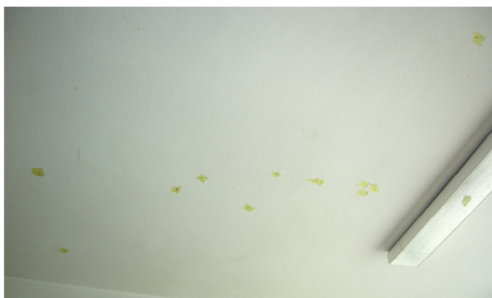
Fig. 5. Points marked on the ceiling at 12.00
