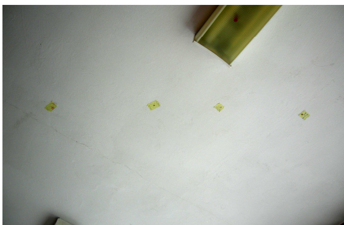
Rys. 6. Points marked on the ceiling at 15.00
