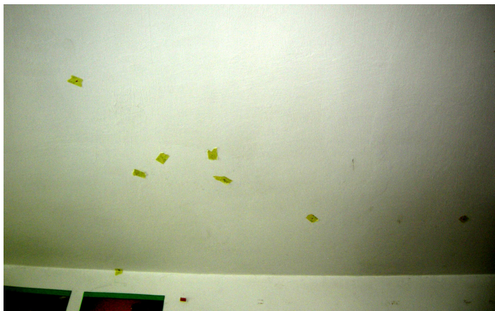
Fig. 4. Points marked on the ceiling at 8.30
