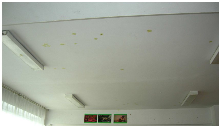
Fig. 1. Picture of ceiling, where the measurement points were marked
